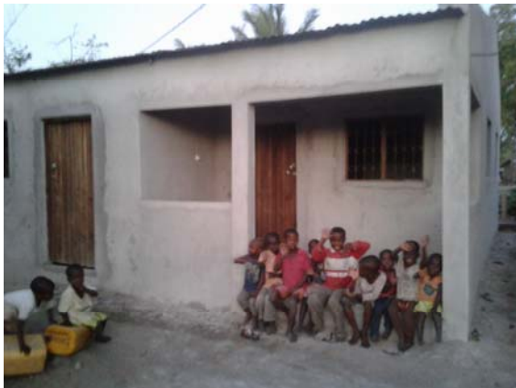
This new building is built on the foundation of the destroyed widow's and very young children's cottage. It will serve the orphans and house the ACPO and MOP church office.
