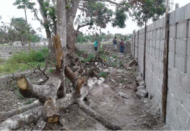
Building a new wall around Tanneken's home.
