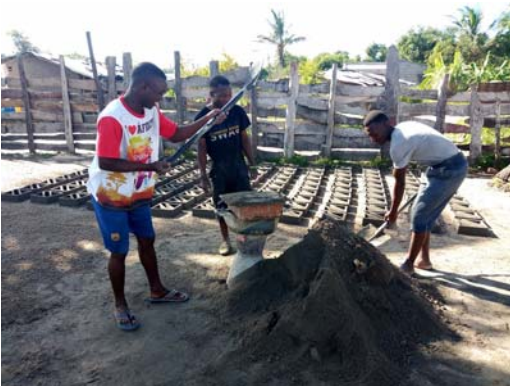
Making cement blocks for the security wall.
